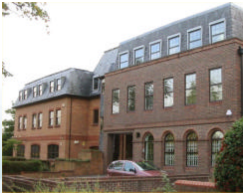
COINS offices in Slough
